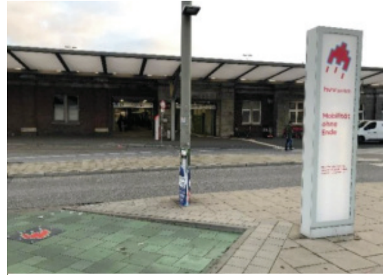
hvv switch Station in Hamburg-Barmbek
